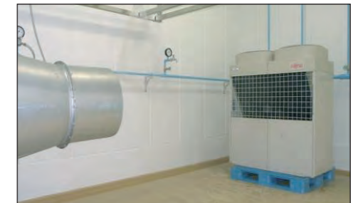
Shower Test Room
