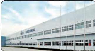
Fujitsu General Central Air Conditioner (Wuxi) Co. Ltd.
