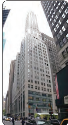
Fujitsu General Solution Centre "THE AIRSTAGE"
