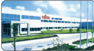
Fujitsu General (Shanghai) Co. Ltd.
